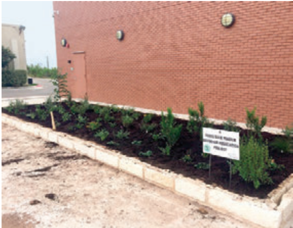
Completed xeriscape planter at the Caldwell County Justice Center. Xeriscape installed here will no need any supplemental from irrigation
