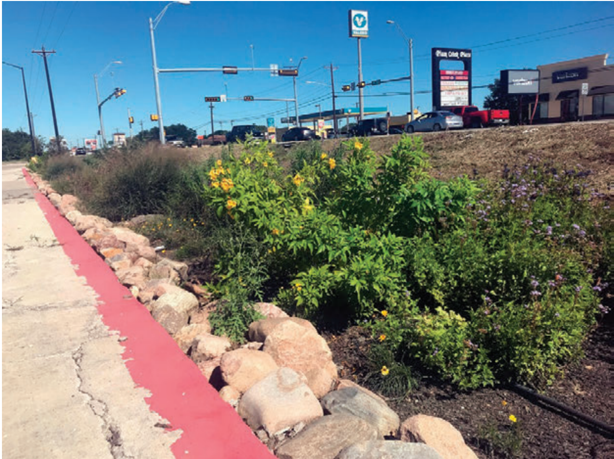
Caldwell County Justice Center rain garden capable of draining and filtering up to 2.26 acres of runoff after completion
