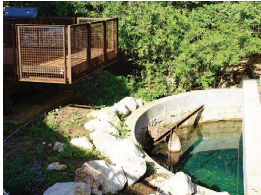
As part of the restoration of the site the Headwaters springs were uncapped, an overlook was installed and interpretive signage created
