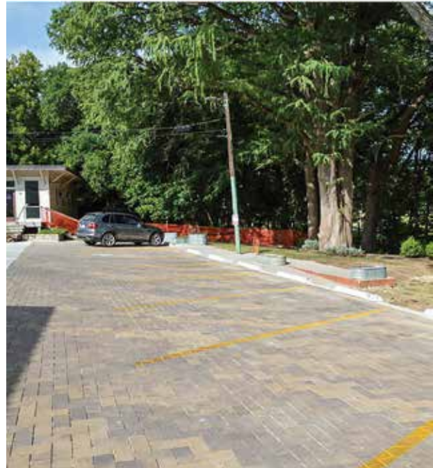
Permeable pavers installed in Downtown Wimberley along a sensitive reach of Cypress Creek.
