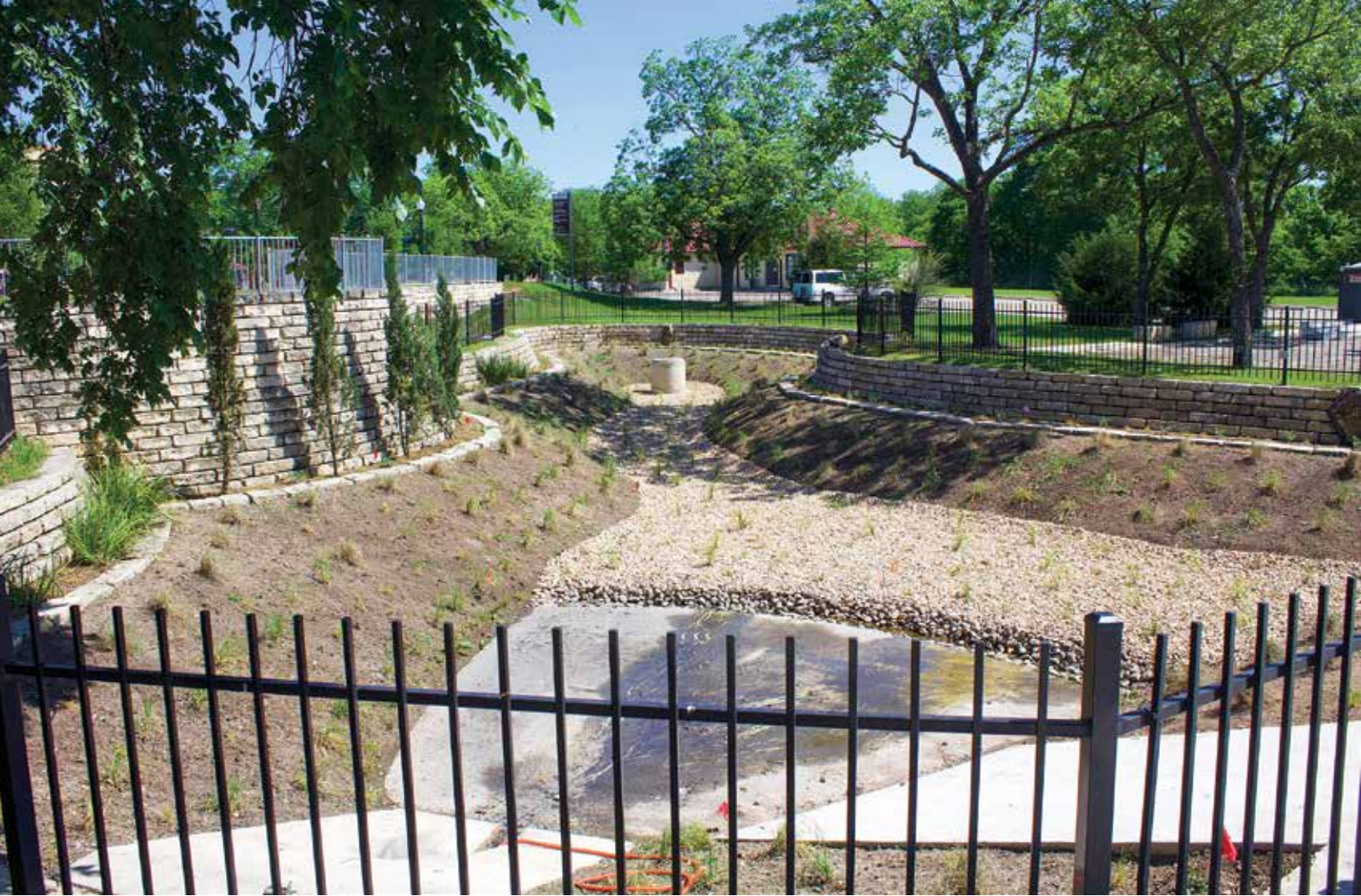
Completed Hutchison biofiltration pond. Photo Courtesy of Aspen Navarro.
