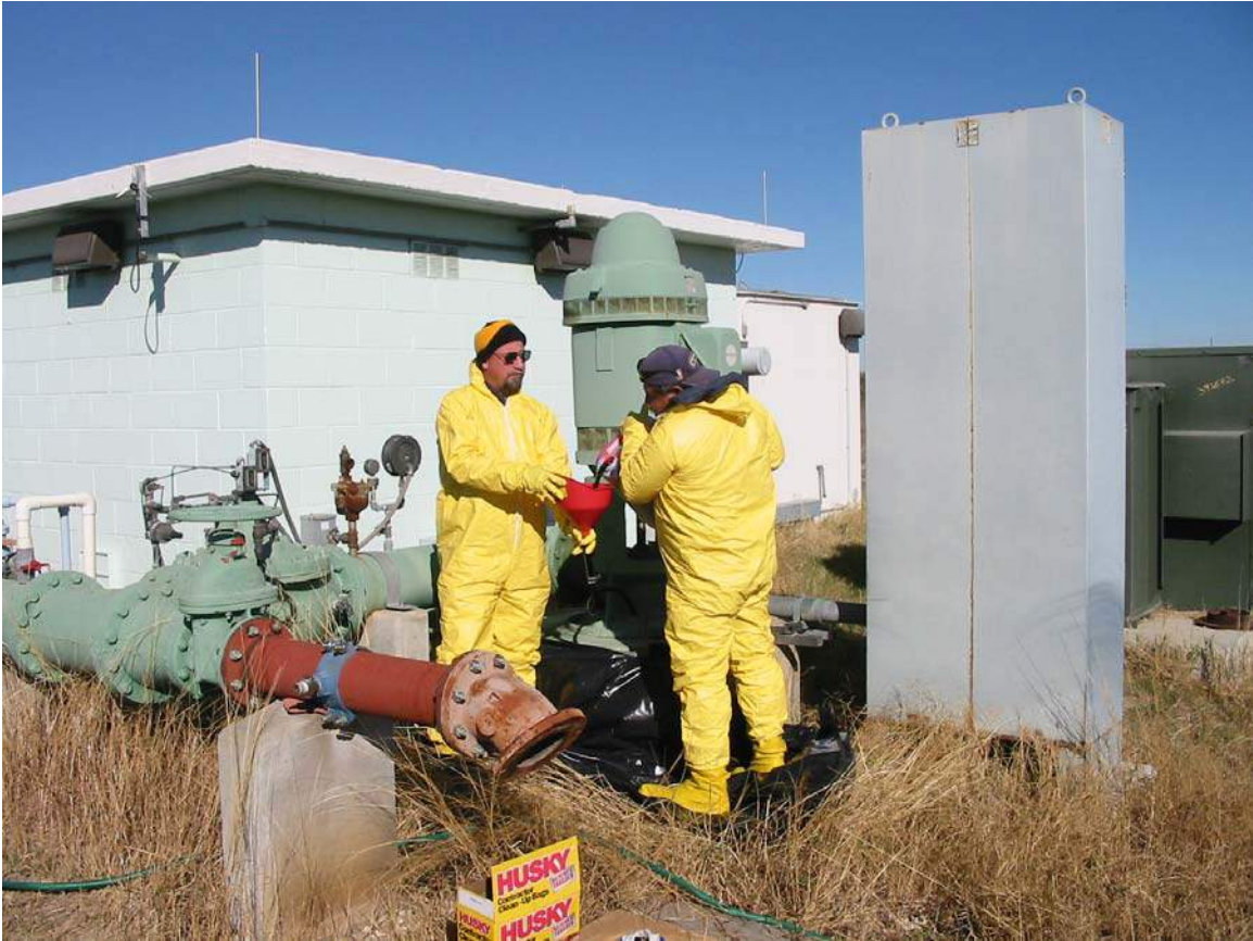
Figure 4.2. Injection of Eosine Dye into Agarita Well on December 11, 2008
