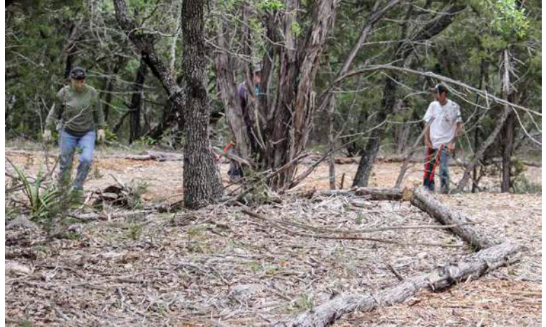
Volunteers work to build trails at the Environmental Learning Center Property adjacent to the Canyon Lake Gorge.
